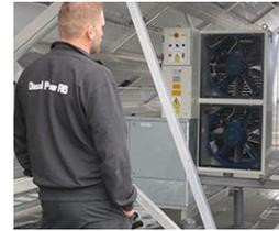
*On the school roof a load bank is installed, which is an electrical load resistance that generates heat energy.*
