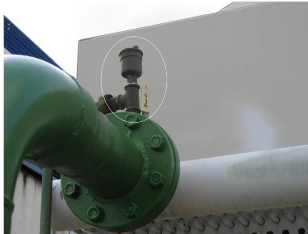
Fig. 3 - Automatic air bleed valve
