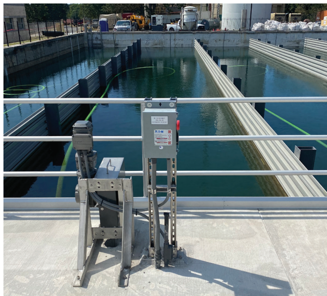
Sedimentation basin at Ozark Point with sludge collection electric motor
