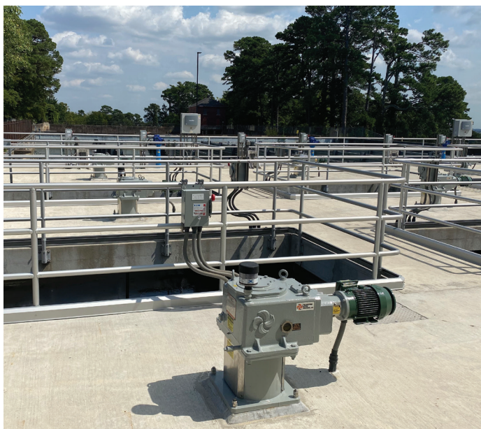
Flocculation basin deck at Ozark Plant with electric mixer motor
