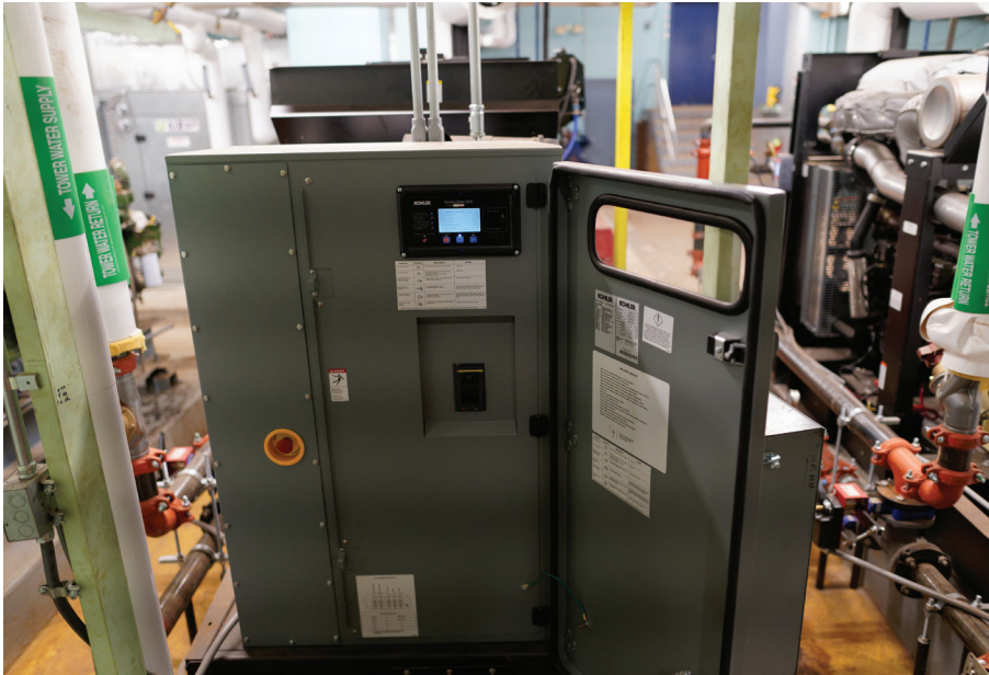
KOHLER. DEC3500 on-board paralleling controller
