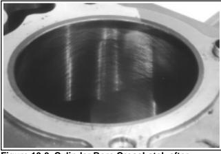
Figure 10-3. Cylinder Bore Crosshatch after Honing.
