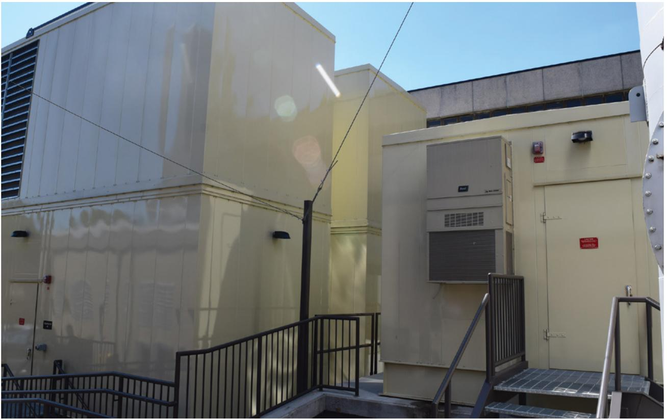
Along with the gen-sets, CK also supplied switchgear and Kohler's Decision-Maker 550 controller designed to provide advanced control, system monitoring and system diagnostics, as well as remote monitoring capabilities.
