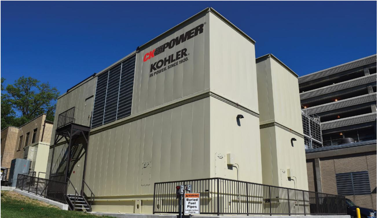
CK Power supplied a pair of Kohler standby diesel generator sets rated 2000 kW each to provide backup power for a new neonatal intensive care unit at SSM Health St. Mary's Hospital in Richmond Heights, Mo. The gen-sets were housed within a custom-designed Chillicothe Metal sound-attenuated enclosure.
